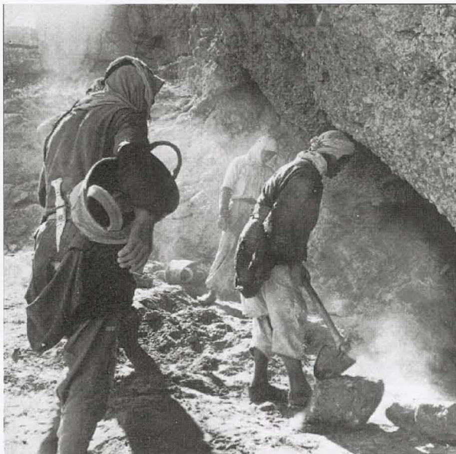
Workers excavate a cave in the limestone cliff.
